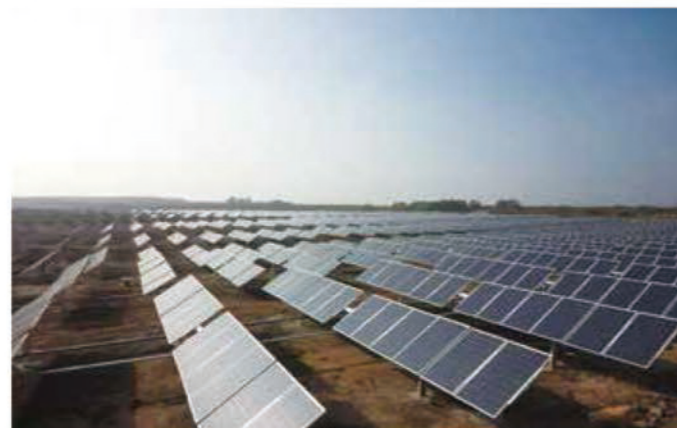
联动式光伏跟踪 Linkage Type PV Tracking
